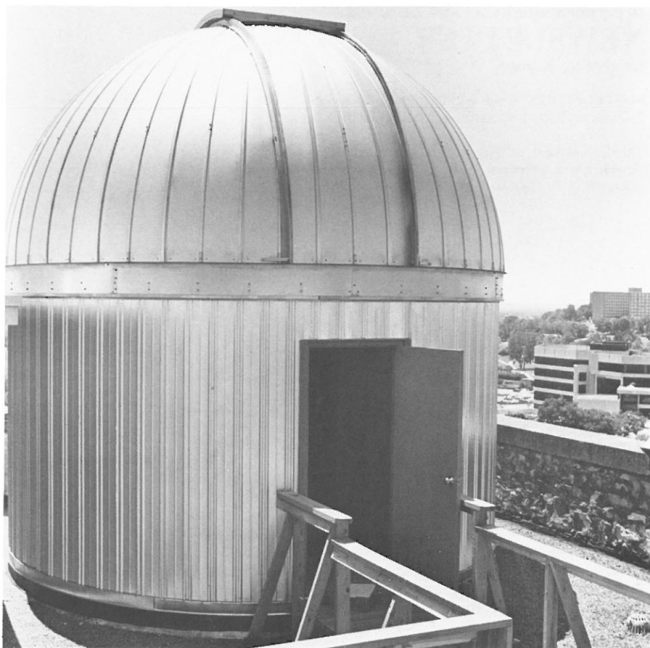
The new sixteen foot Ash Dome and wall cylinder houses the 6-inch Clark refractor. Installation was completed in early June, five years after the old structure was condemned as unsafe. This Ash dome is fully electrical.
